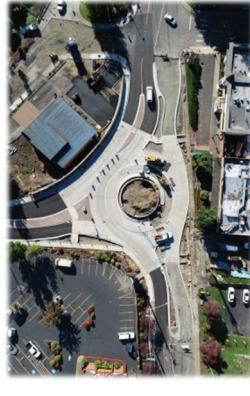
LaCenter Rd / 4th St Roundabout
