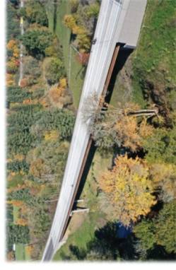
NE 10th Ave Bridge Project
