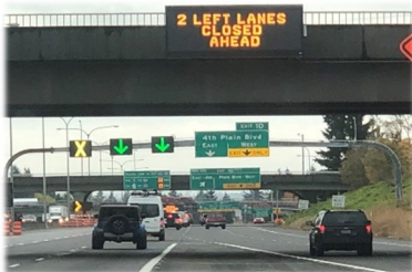
I-5 Advanced Traffic Management System
