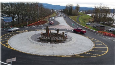
SR-14 Roundabouts in Washougal
