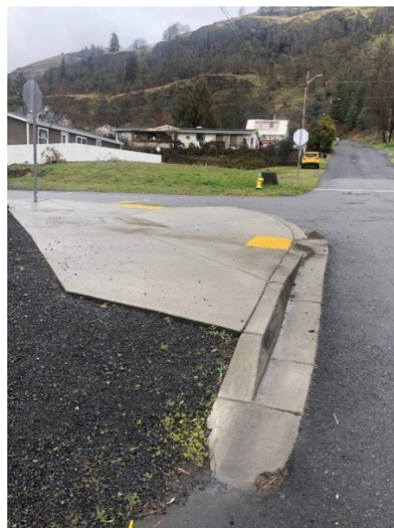
Ramp, southwest corner of Cedar and Steuben, completed as part of another project
