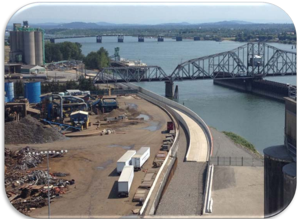
Rail Trench, Port of Vancouver
