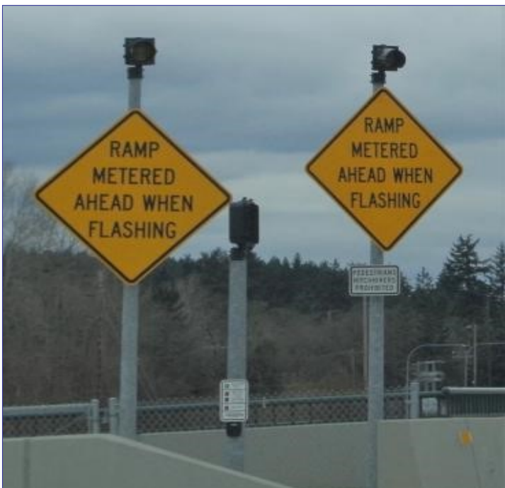
Ramp Meter Warning Signs
