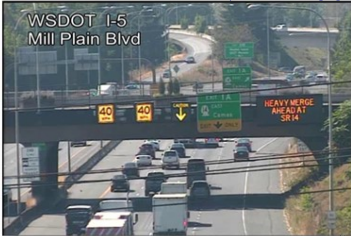
Camera view, variable speed and warning signs
