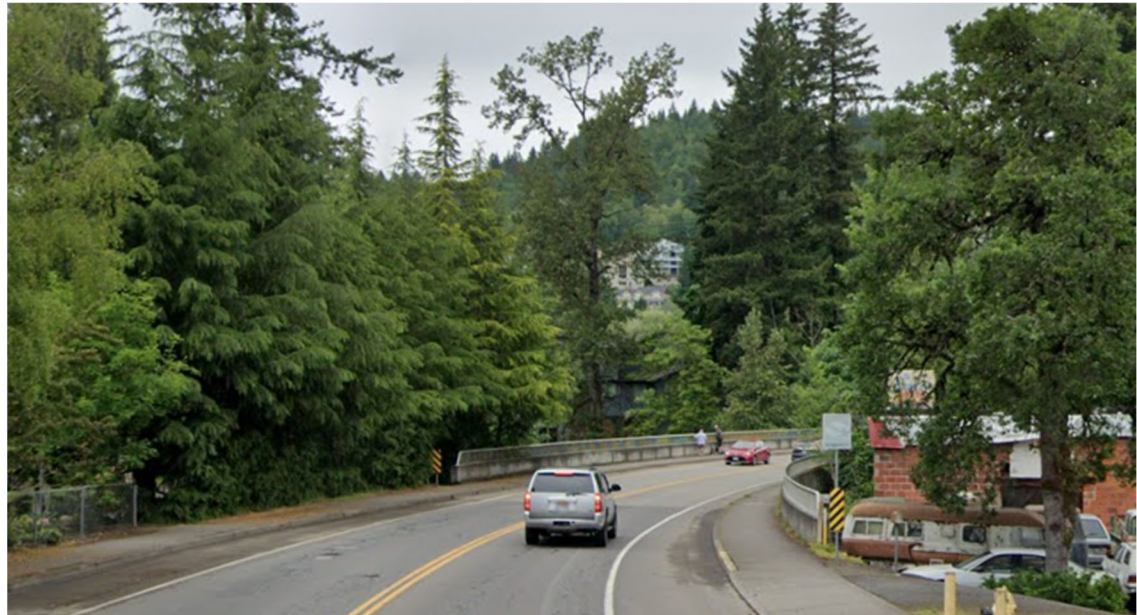
Figure 9. Facing northbound on Washougal River Road and approaching bridge crossing.
